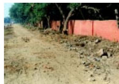
Construction of peripheral road
