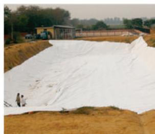
Geomembrane sheet lined water reservoir
