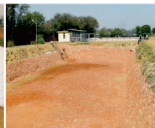
Geomembrane sheet covered with bricks
